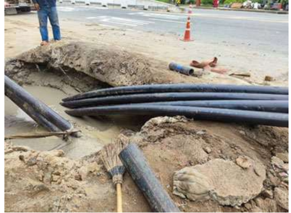
TRUE Horizontal Directional Drills (HDD) / Satun
