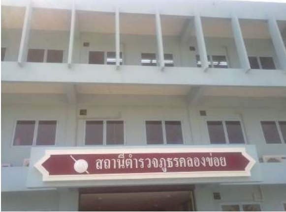
Khlong Khoi Police Station - Nonthaburi
